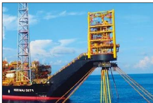
Figura 1. Torreta externa. ( https://hvac4offshorevn.wordpress.com/ )
