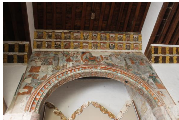
Fig. 5. Arco principal interior
