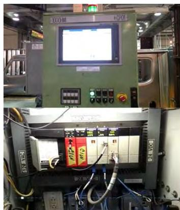
Figura 2. PLC y software RS Logix 5000
